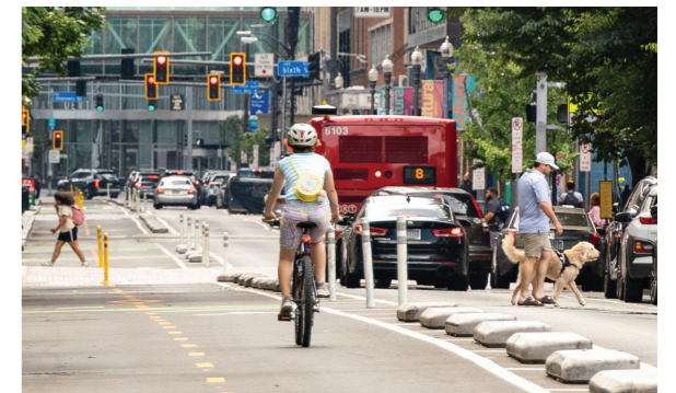
This image shows the protected bicycle infrastructure on Penn Avenue in the Strip District, which is similar to the bicycle infrastructure that will be placed on Fifth Avenue in Oakland.
